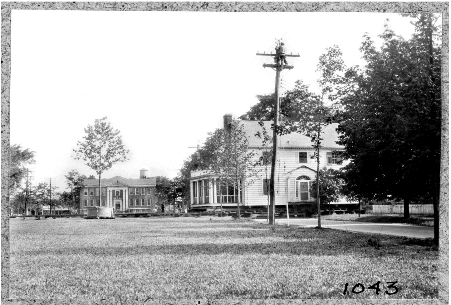
The Bathurst-Peachy House being moved across Palace Green, Williamsburg, Virginia, circa 1930. In the background, the old Williamsburg High School is shown prior to its demolition. Photo by Susan Higginson Nash .
