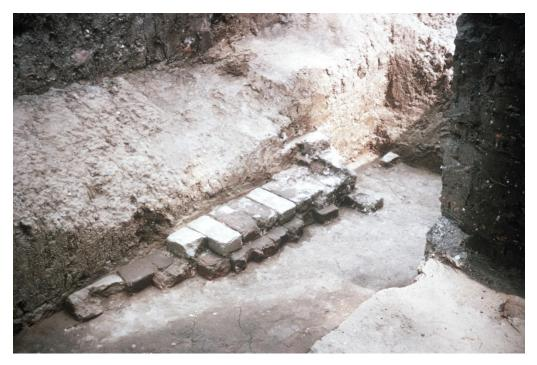
Figure 6: Surviving section of foundation within the cellar.
